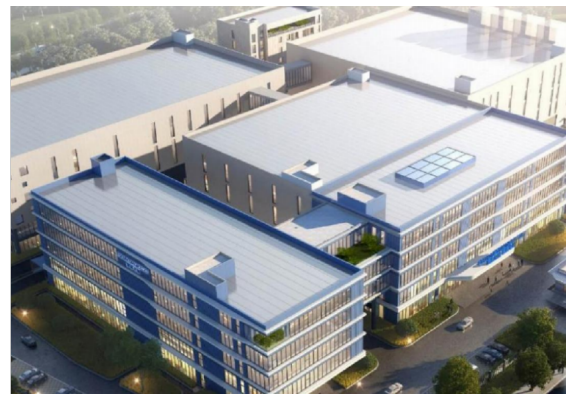
Fosun Diagnostics Second Headquarters
